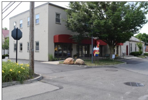
37 W Bridge St, looking northwest
