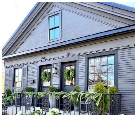
After, Iron Ore
