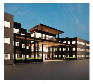
with a metal and glass railing. The remainder of the structure is an elevated canopy with slatted wood panels. The soffits of the canopy and building addition will be constructed of metal panels
