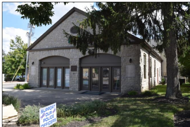
37 W Bridge St, looking southeast
