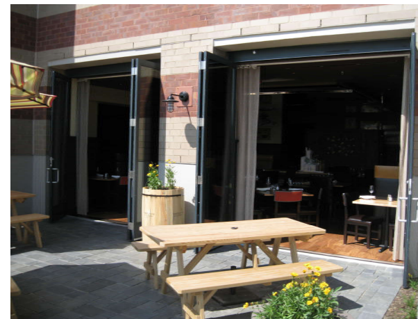
Ramco (or equal) Operable Folding Wall System, finish to match building standard
