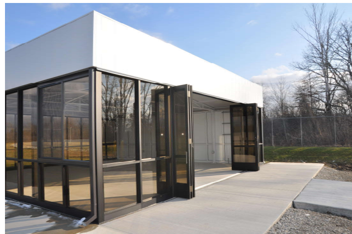
Ramco (or equal) Operable Folding Wall System, Finish to match building standard
