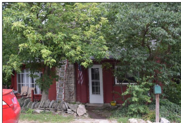
62 N Riverview St, looking northeast
