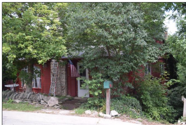
62 N Riverview St, looking southeast
