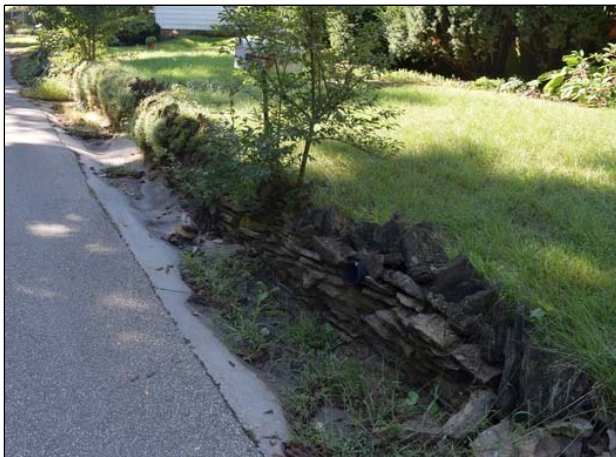
Overview of wall, looking south
