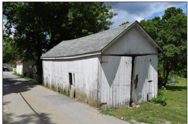
45 N Riverview St, ancillary structure, looking northeast
