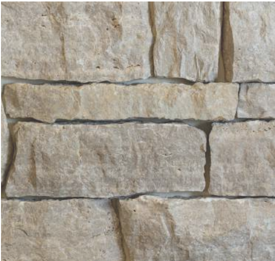
Limestone veneer over foundation and exterior wall
