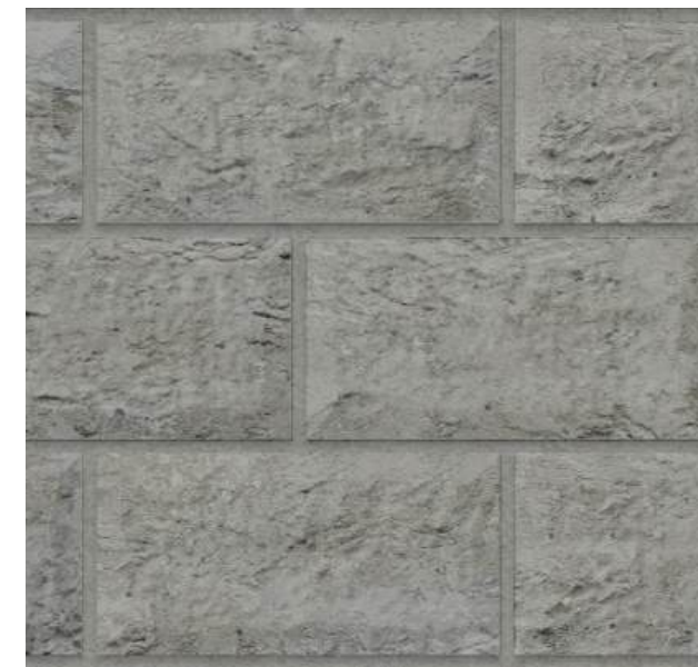
6. Rough Concrete Rockface to match Existing Stone
