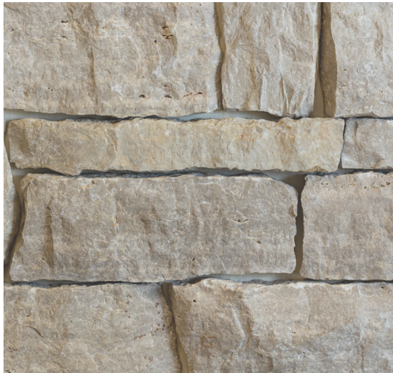
Limestone veneer over foundation and exterior wall
