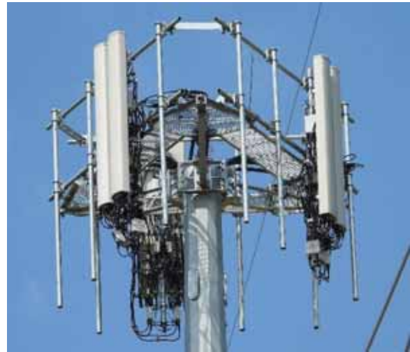
Photo 2: Triangular Platform with Verizon Antennas
