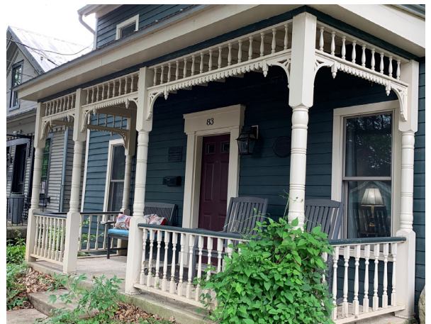
Porch, 83 South High Street
