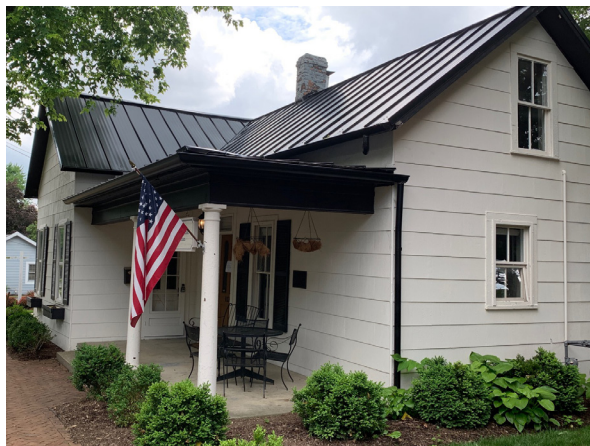
Historic building color, 113 South High Street
