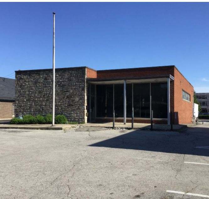
Former Post Office at 38 West Bridge Street, built in 1965, is in a Modernist Movement architectural style. The one-story brick and stone building has a rectilinear footprint with flat roof and a large glazed storefront window.
