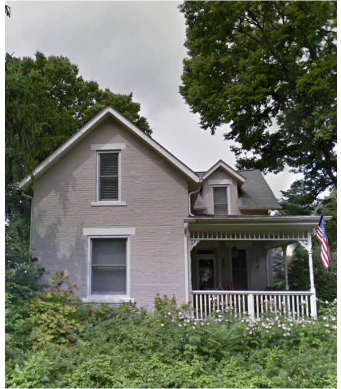
55 South Riverview Street, built ca. 1900, is an example of the Gabled Ell building type with No Academic Style. The front block and wing are identifying forms with the spindle work suggesting an increased accessibility of millwork at the turn of the century.
