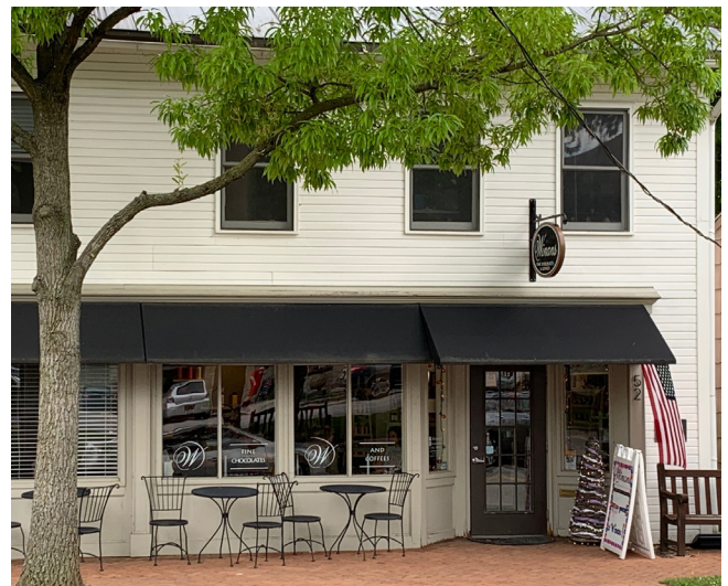
Recessed entry and bulkheads, 52 South High Street
