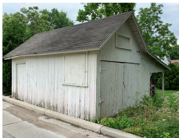
Historic outbuilding, 83 South Riverview Street
