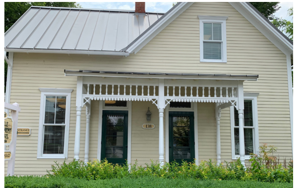
Original architectural details, 138 South High Street
