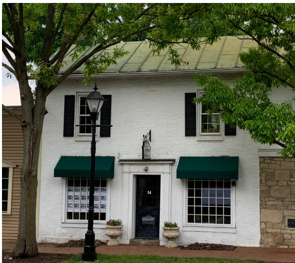
Commercial storefront, 14 South High Street
