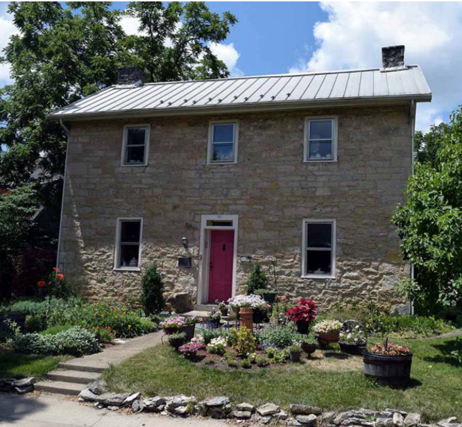
83 South Riverview Street, built in 1824, is an example of an I-House building type with Federal architectural style elements. The building is of stone construction with a standing seam metal roof.
