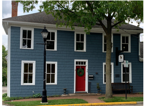
Historic building color, 76-78 South High Street
