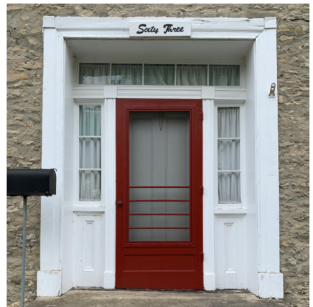
Original storm door, 63 South High Street
