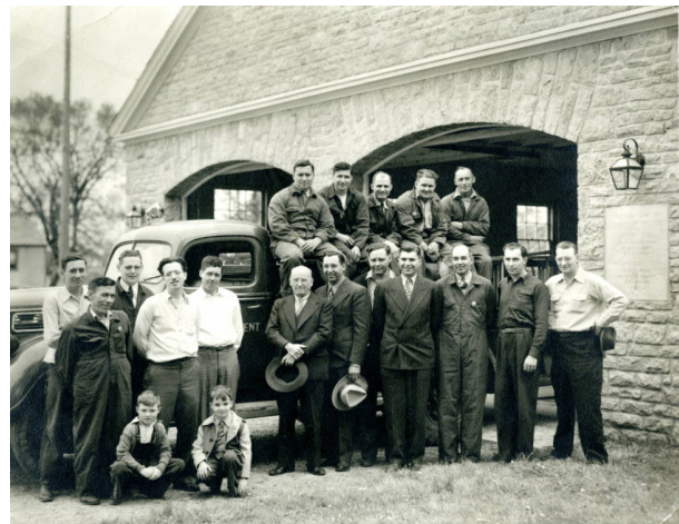
Dublin Firehouse, 37 West Bridge Street, 1945
