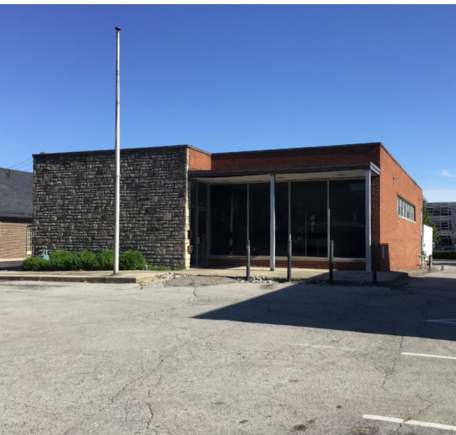
Former Post Office at 38 West Bridge Street, built in 1965, is in a Modernist Movement architectural style. The one-story brick and stone building has a rectilinear footprint with flat roof and a large glazed storefront window.
