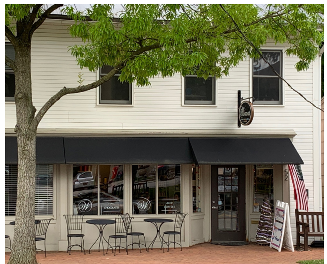
Recessed entry and bulkheads, 52 South High Street
