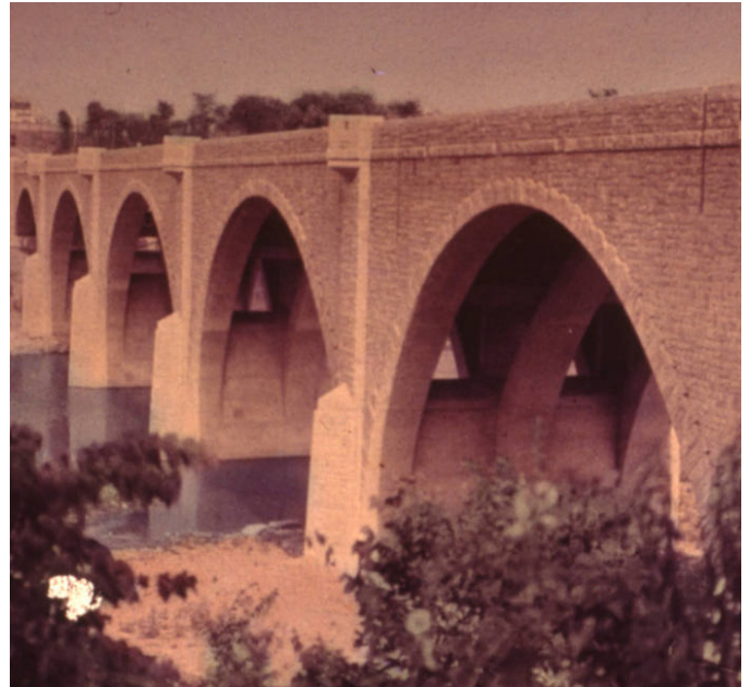
Bridge Street Bridge, 1935
