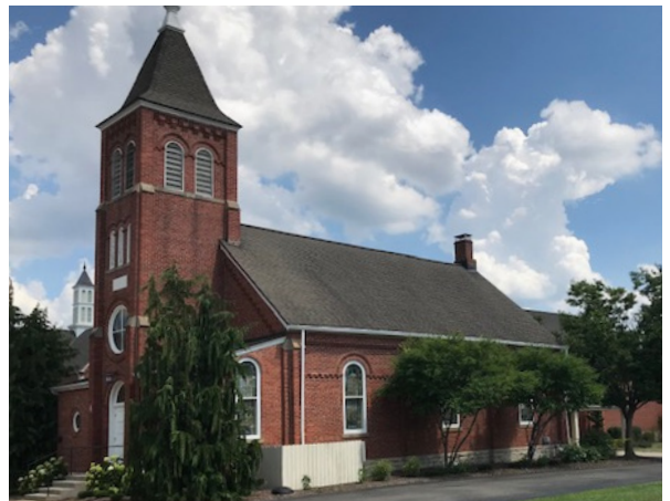
St. John Lutheran Church, 6115/6135 Rings Road
