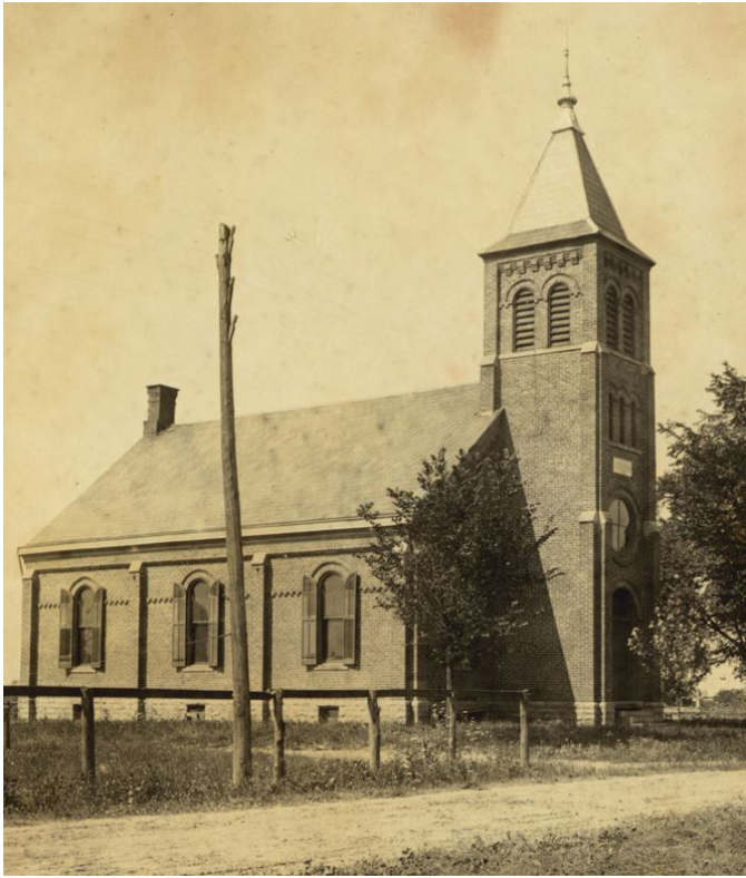
St. John Lutheran Church at 6135 (6115) Rings Road, built ca. 1860, is an example of Romanesque Revival architecture. Note the elements such as the masonry construction, round arches, brick corbeling, and square tower.
