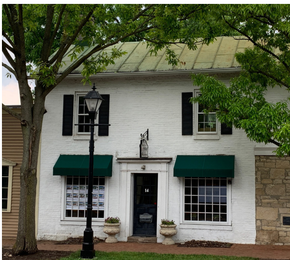
Commercial storefront, 14 South High Street
