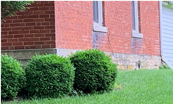
Original stone foundation, 167 South High Street
