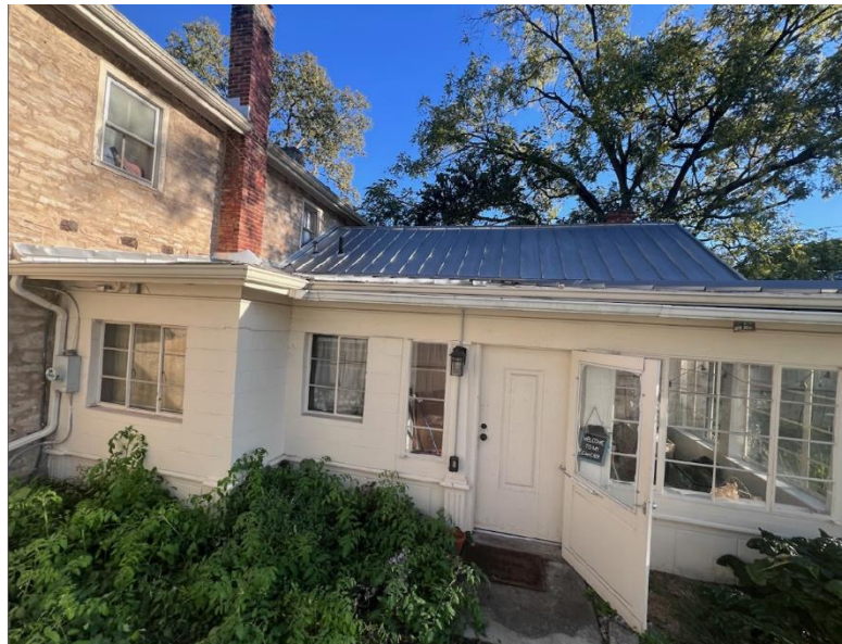
Porch and chimney to be removed
