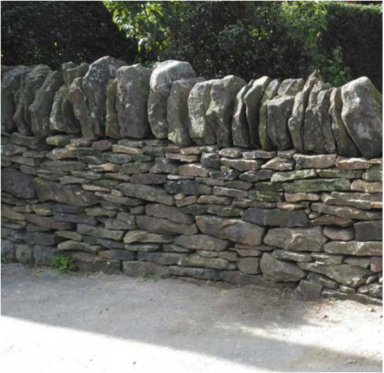
Reconstructed historic stone wall (see landscape plans for more information)
