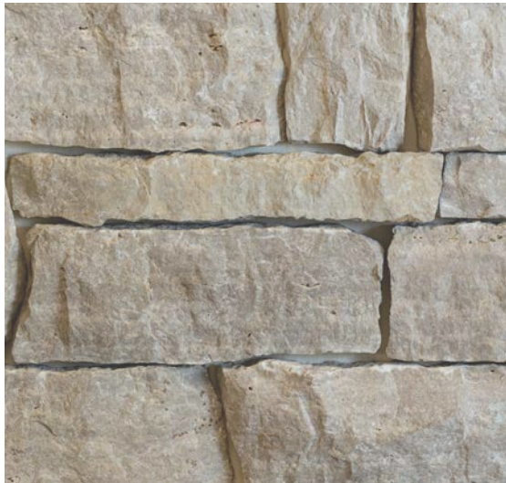
4. Limestone veneer over columns and partial foundation
