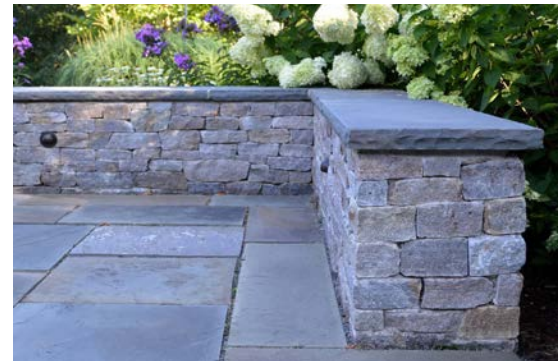
limestone wall with cast stone cap (see landscape plans for more information)
