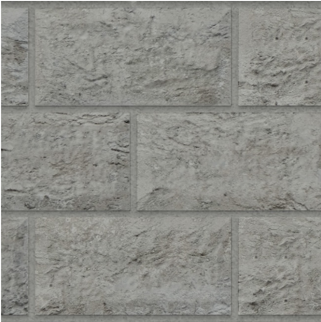
4. Classic Rock Face Block #201 - cast concrete veneer over CMU
