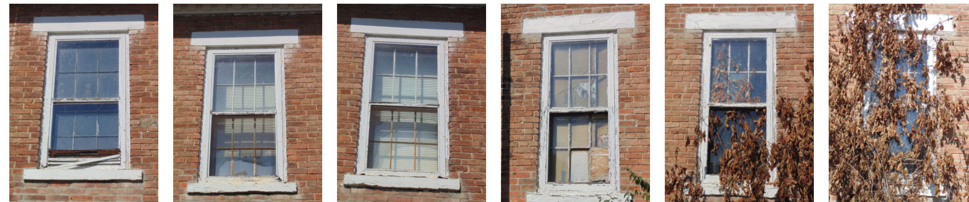
WINDOW 15 WINDOW 14 WINDOW 13 WINDOW 12 WINDOW 11 WINDOW 10
