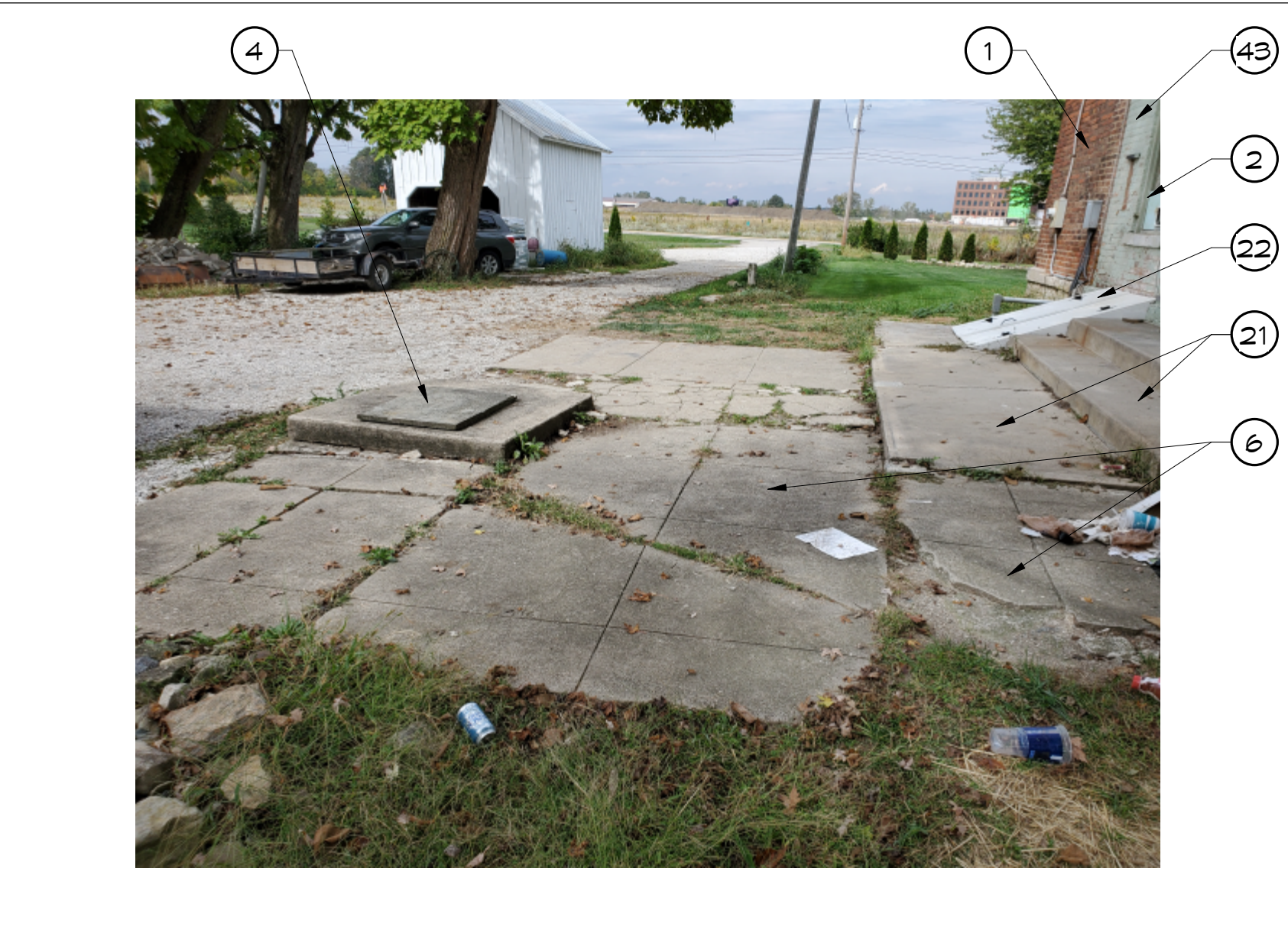
(WEST) EXISTING CONCRETE PAVING
