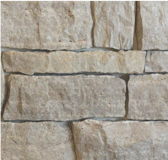
Limestone veneer over columns and partial foundation
