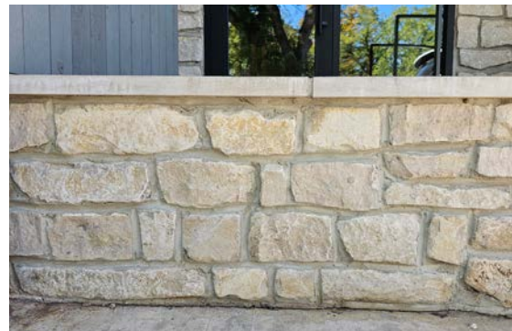
Stone wall with cast stone cap
