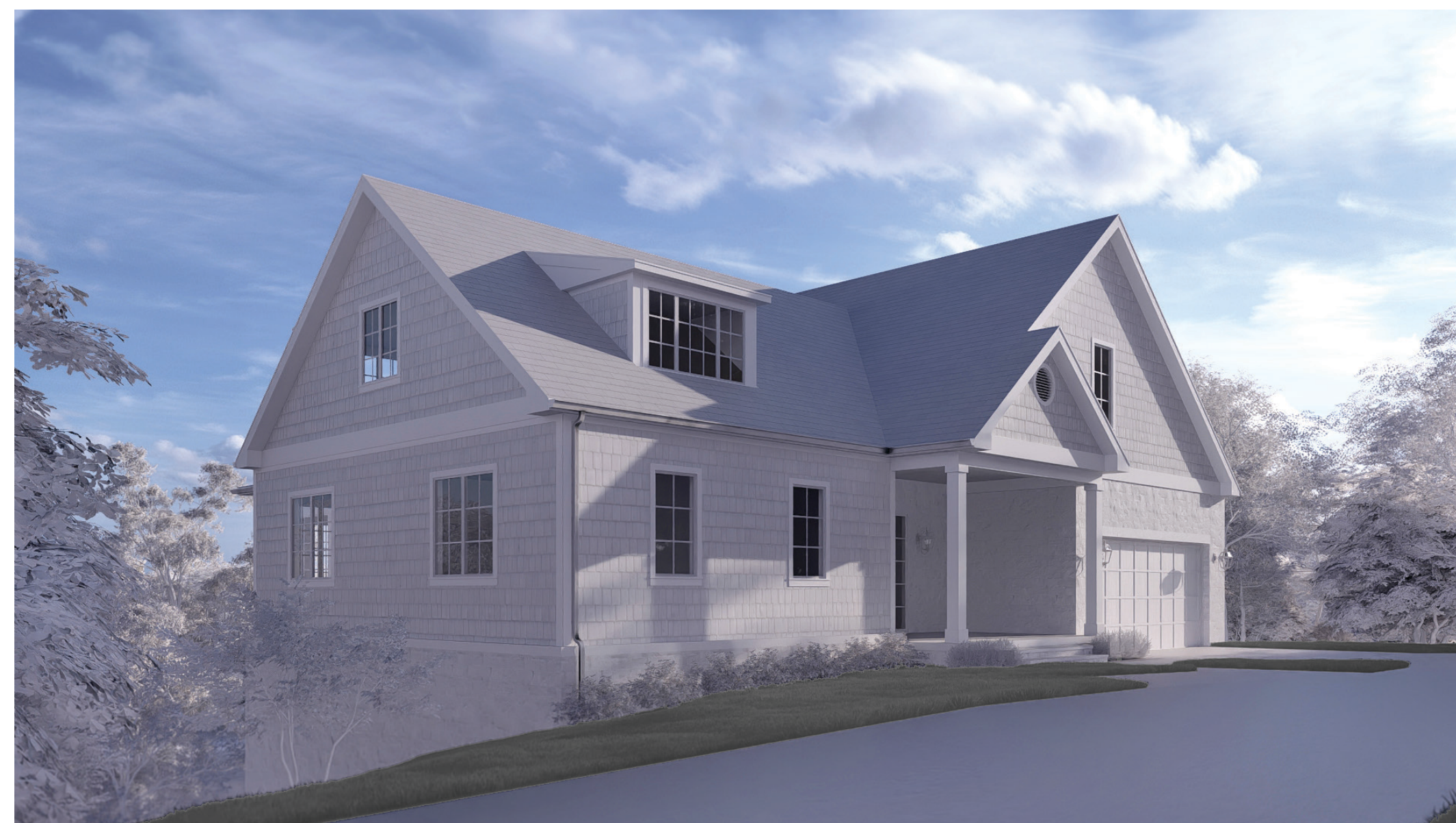
NORTH FACADE VIEWED FROM S. RIVERVIEW ST
