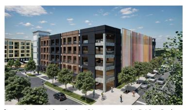
permitted to include parking on the roof, consistent with other parking garages in Bridge Park. The garage is proposed to be clad in brick, cast stone, and storefront systems with a perforated aluminum scrim on the south facade that will incorporate artwork in the future.
