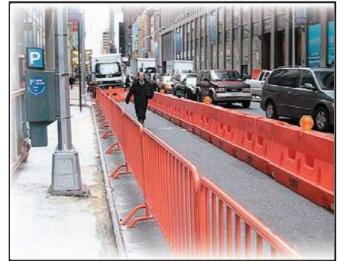
Temporary Pedestrian Walkway
