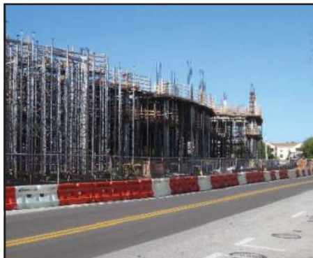
Longitudinal Channelizing Barricade
