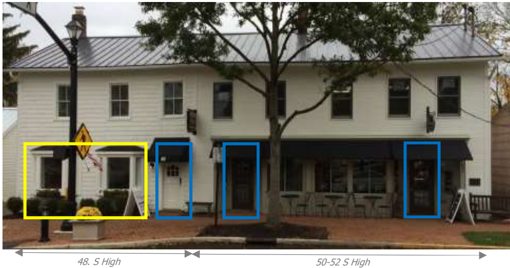
Existing Street View
