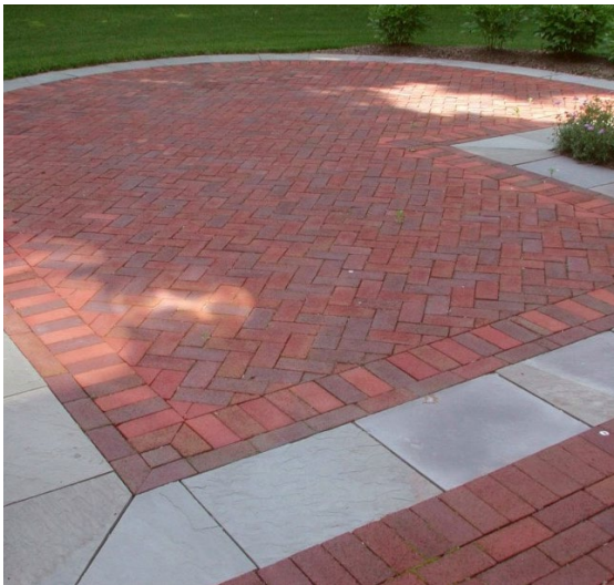
Flush Limestone border to match step tread (see landscape plans for more information)
