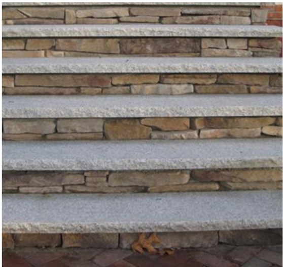
Step with Limestone Tread and Stone Veneer Riser (see landscape plans for more information)
