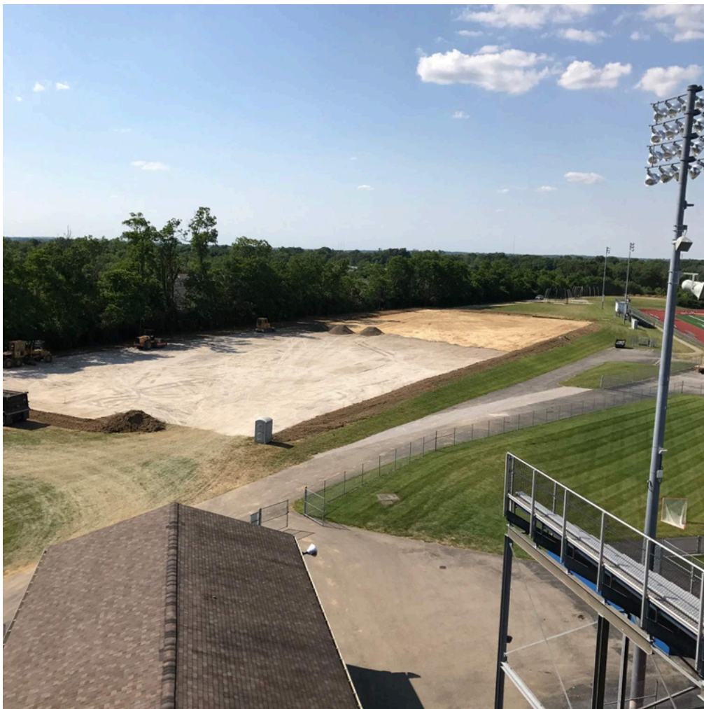
Stone installation & compaction
