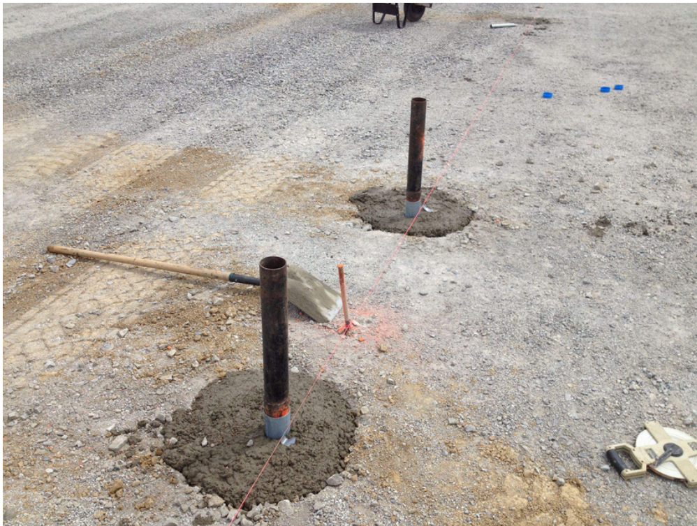
Net post footer installation.
