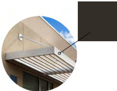
(N) CANOPY (CUSTOM) STYLE: HANGER-SUPPORTED SUNSHADES FRAME: METAL, DARK BRONZE PROFILE: CUSTOM
