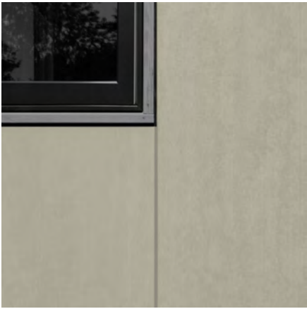
(C) FC-1 FIBER CEMENT TRIM & PANEL JAMES HARDIE COBBLE STONE SMOOTH
