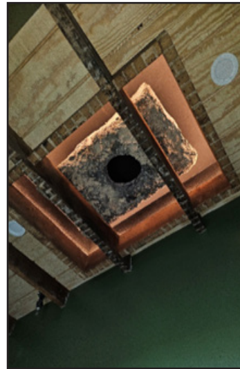
Original Chimney Flue Collar
