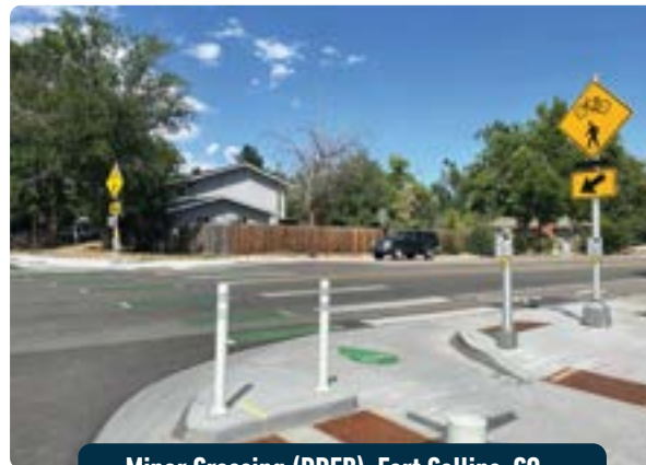
Minor Crossing (RRFB), Fort Collins, CO
