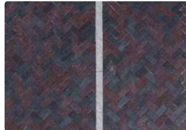
Dark brick herringbone paving to use as a trail surface in the identified Urban areas
