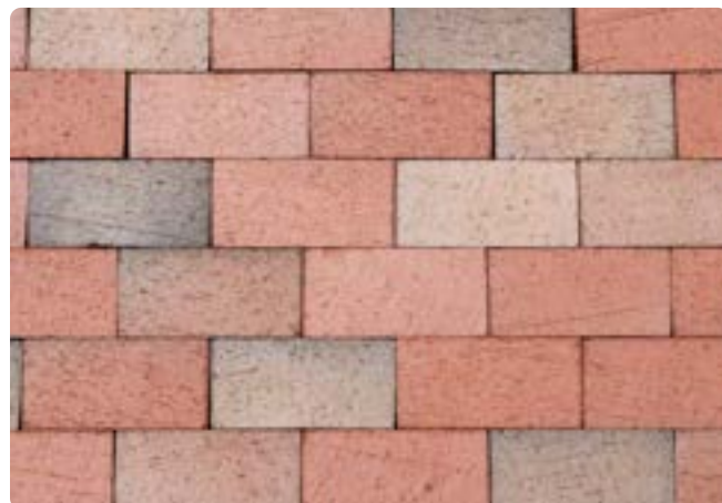
Stack bond brick paving for the amenity zone along the trail
