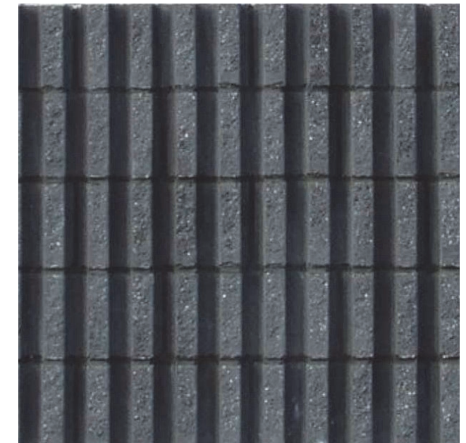
SPLIT RIB BLOCK MASONRY
