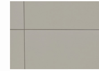
FIBER-3 JAMES HARDIE SMOOTH HARDIE PANEL PAINTED SW7030 ANEW GRAY
