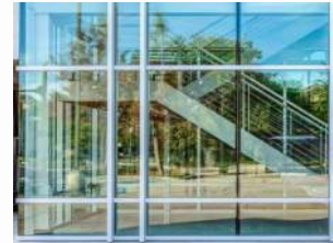
STOREFRONT TUBELITE ALUMINUM STOREFRONT IN BLACK WITH VIRACON VRE 1-59 #2 SURFACE
