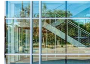
STOREFRONT TUBELITE ALUMINUM STOREFRONT IN BLACK WITH VIRACON VRE 1-59 #2 SURFACE
