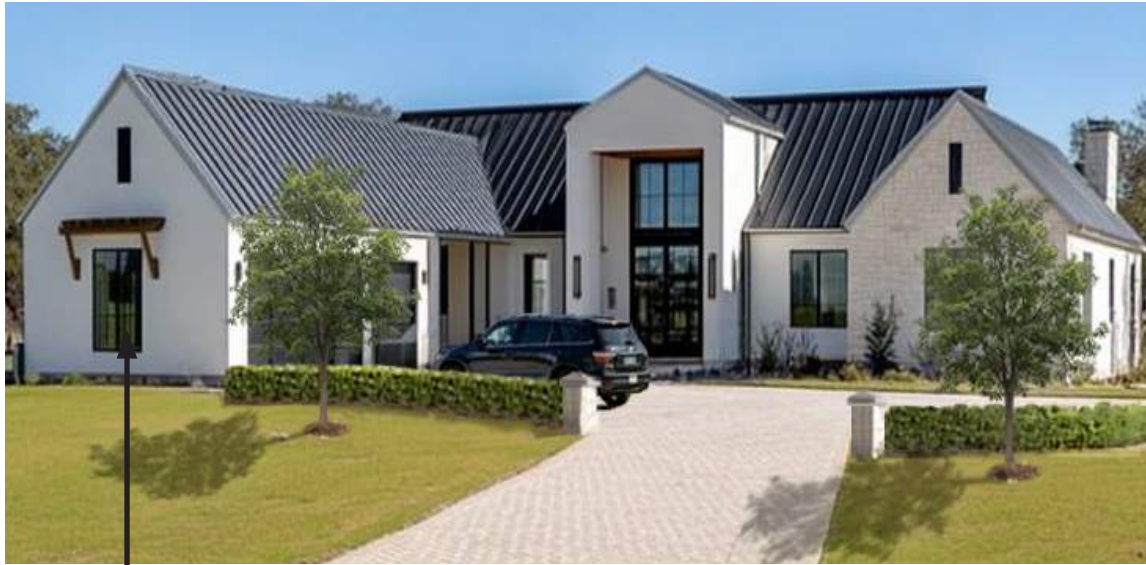
COURTYARD RANCH | 1.5 STORY FACADE WITH DECORATIVE ARCHITECTURAL FEATURE
