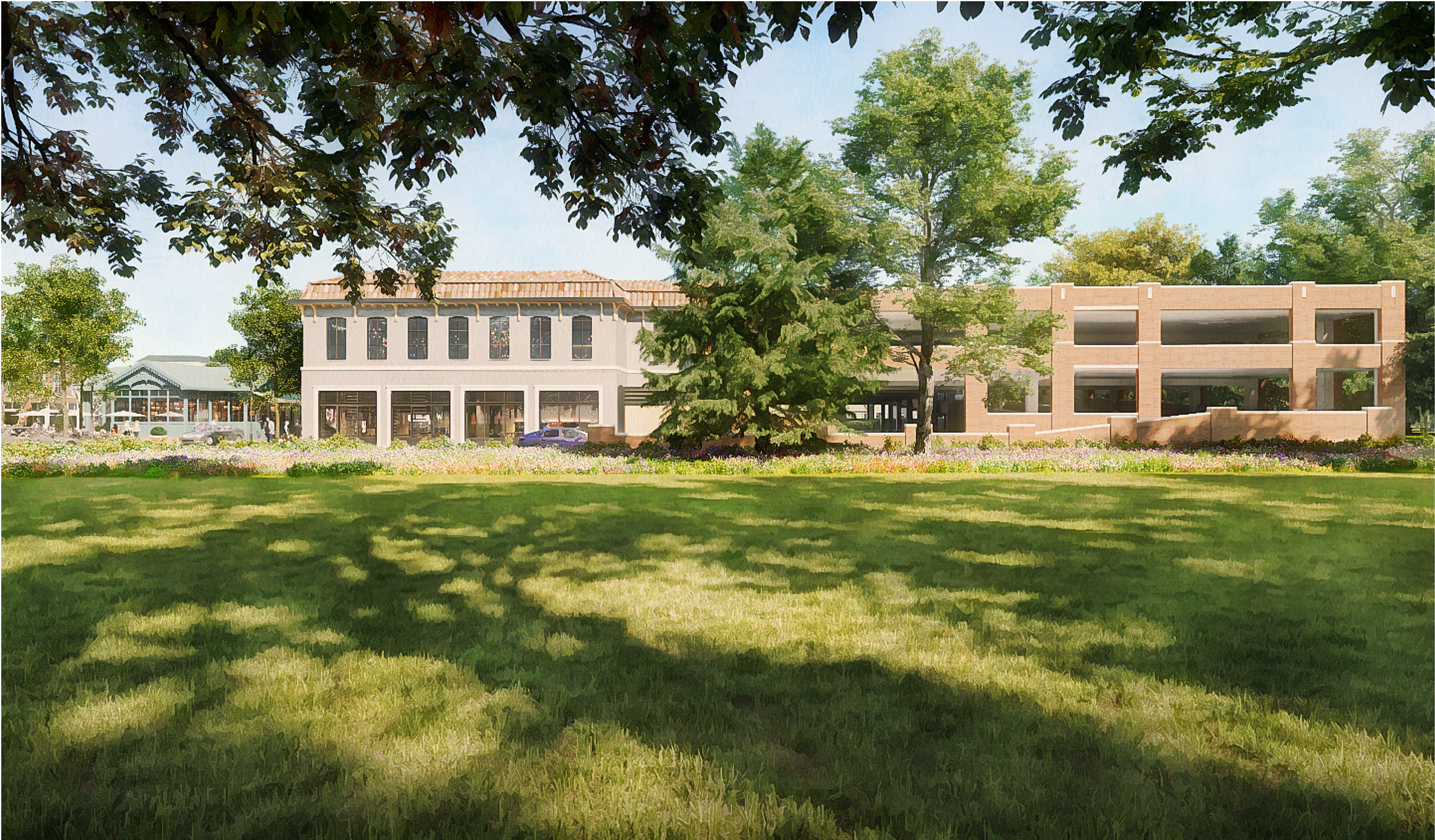
VIEW LOOKING NORTH TOWARD BUILDING G & GARAGE
