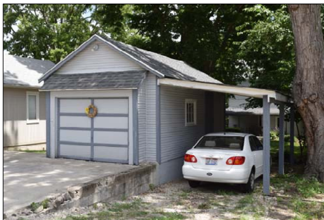
61 S Riverview St, looking northeast
