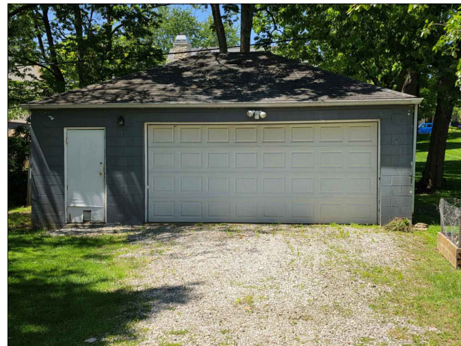
existing garage before
