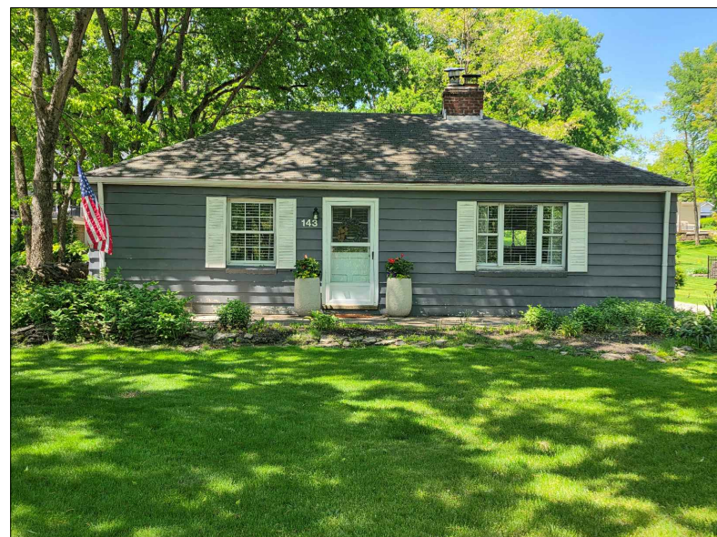
existing home before
