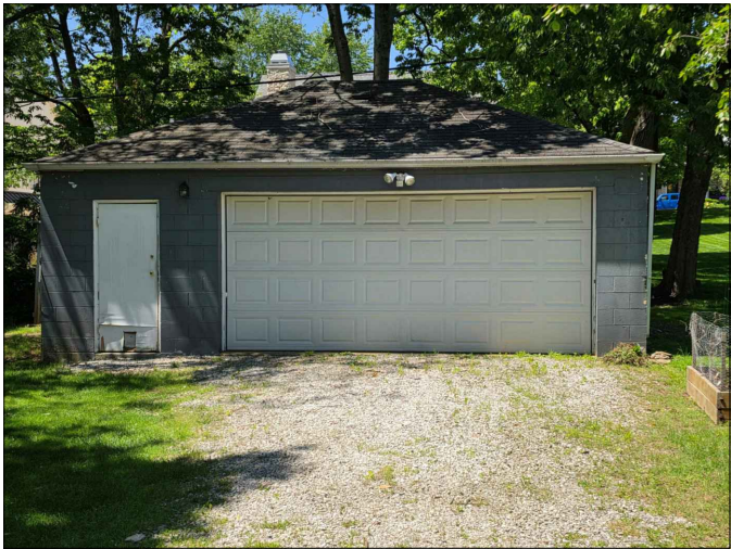
existing garage before
