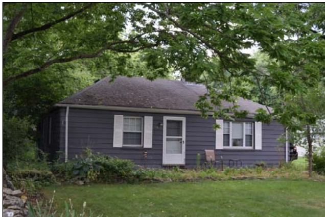
143 S Riverview St, looking northwest
