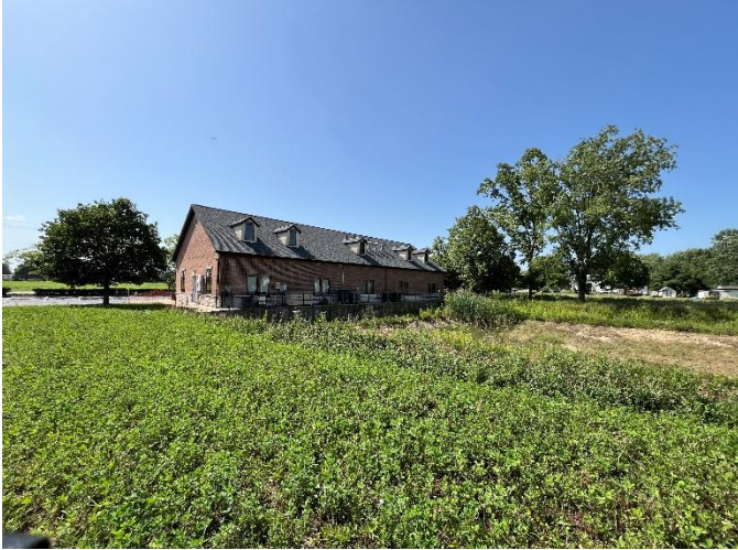
Figure 1 - Existing medical office building on subject property (SO)
