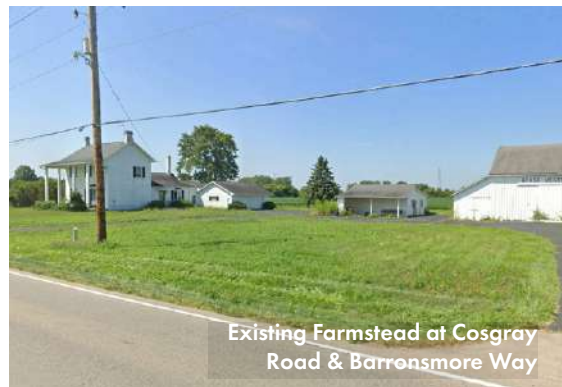
Existing Jewett Farmstead on Cosgray Road
