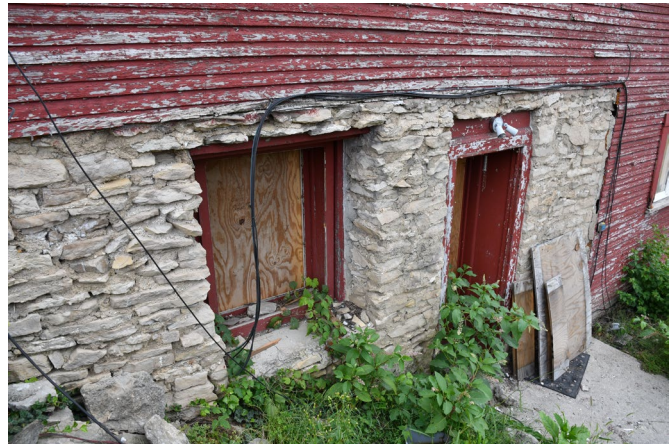
Stone Foundation Wall
