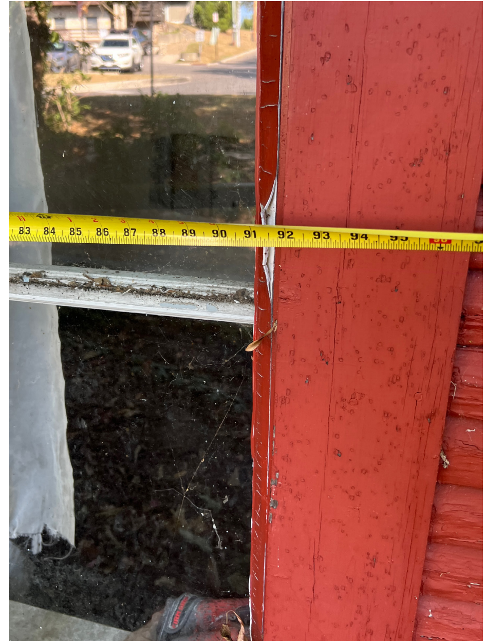
West Arch Window Jamb to NW Corner
