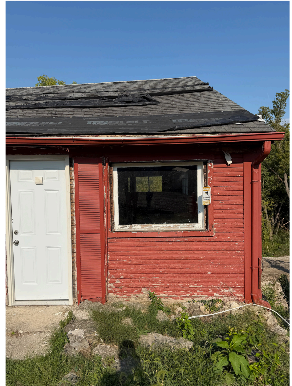
South end of West Elevation
