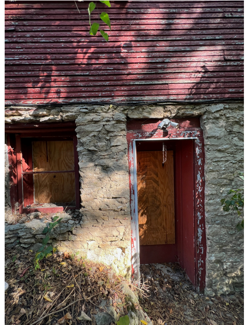
South Door Detail
