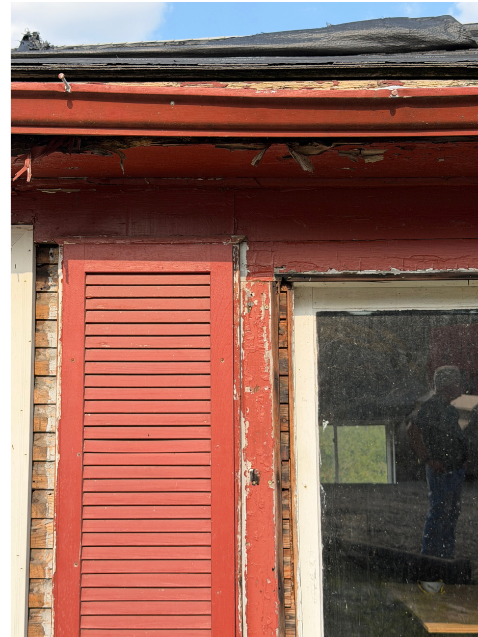
West Window Trim and Shutter Detail
