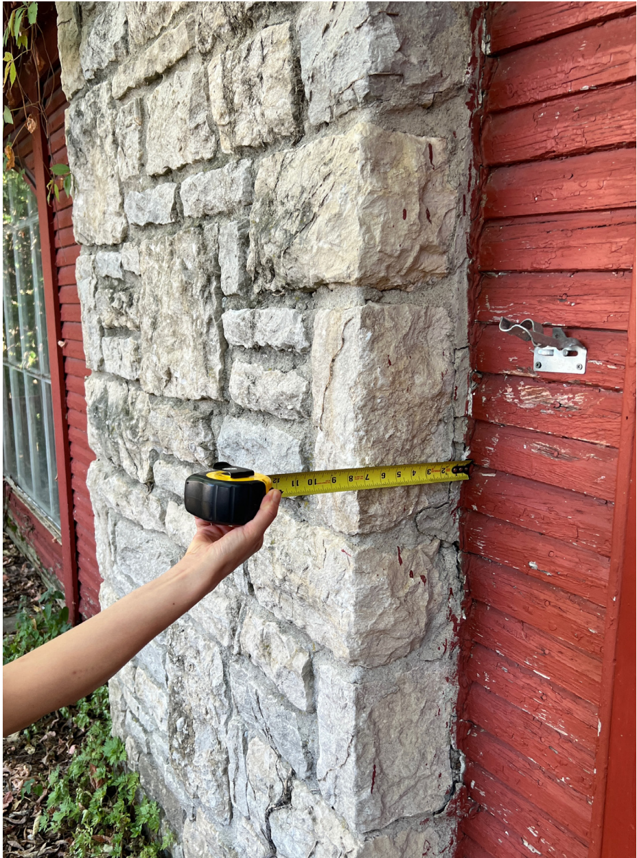
West Chimney Projection
