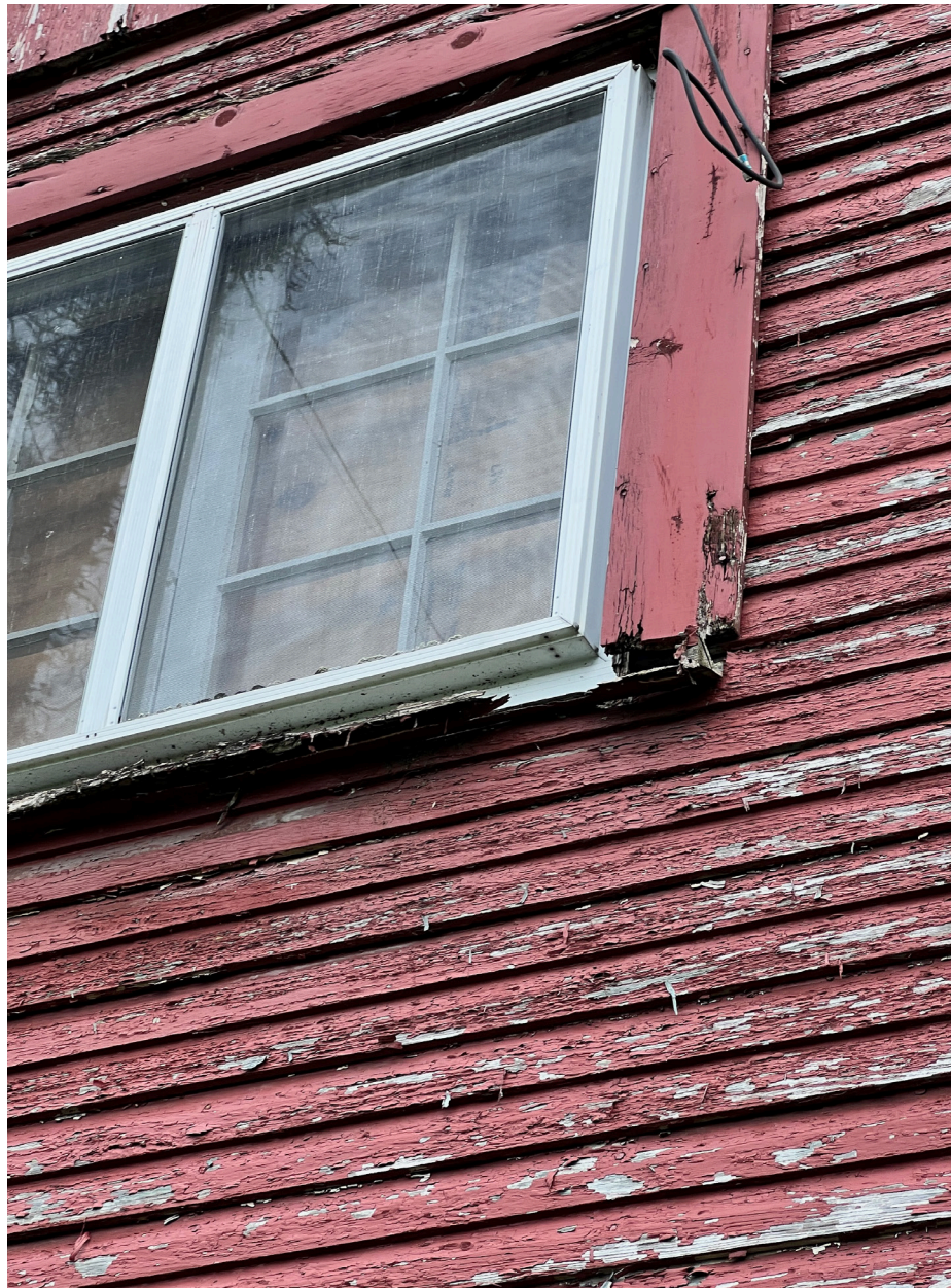
South Upper Window on West
