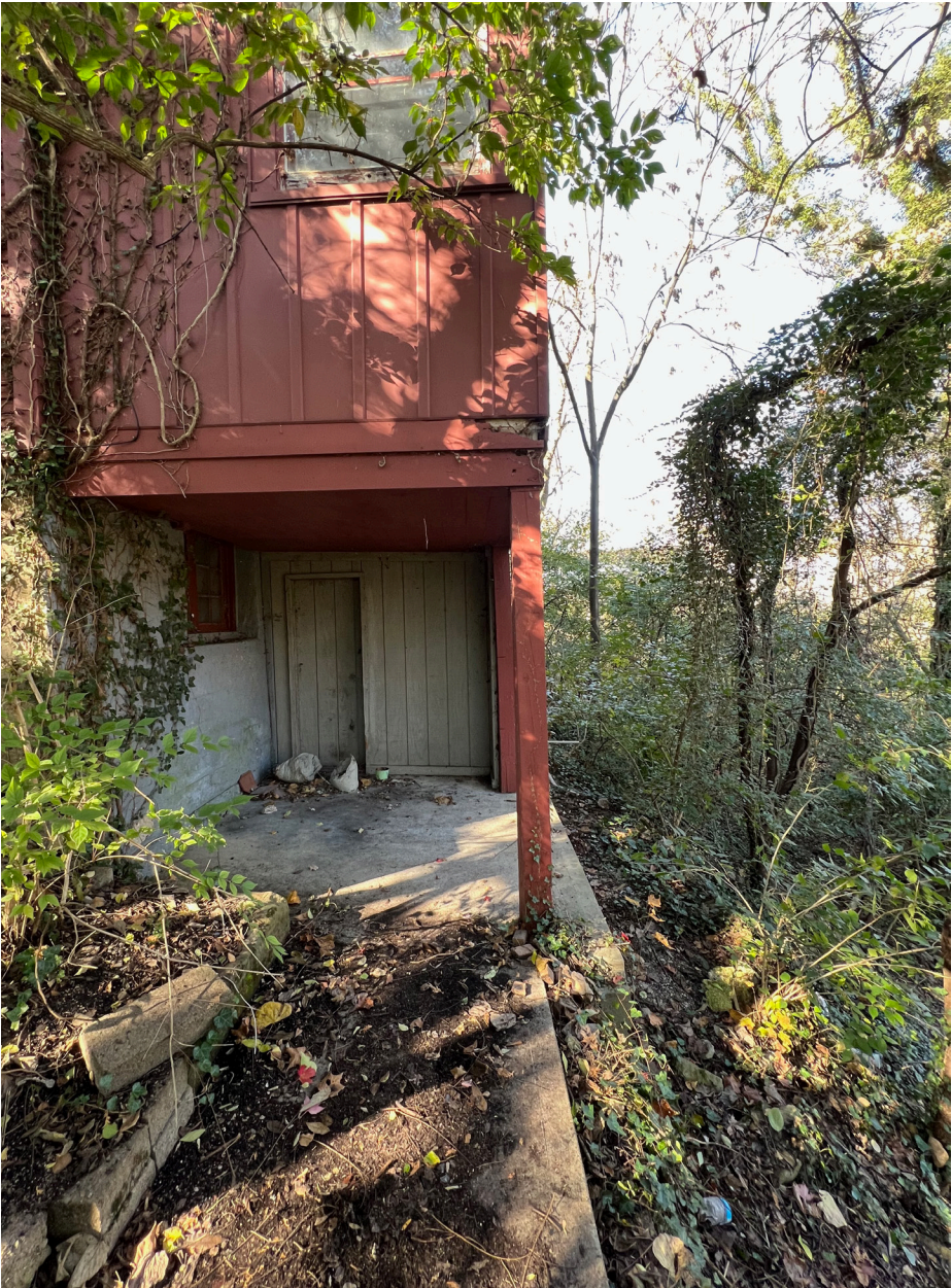
South Partial Elevation near the East Corner
