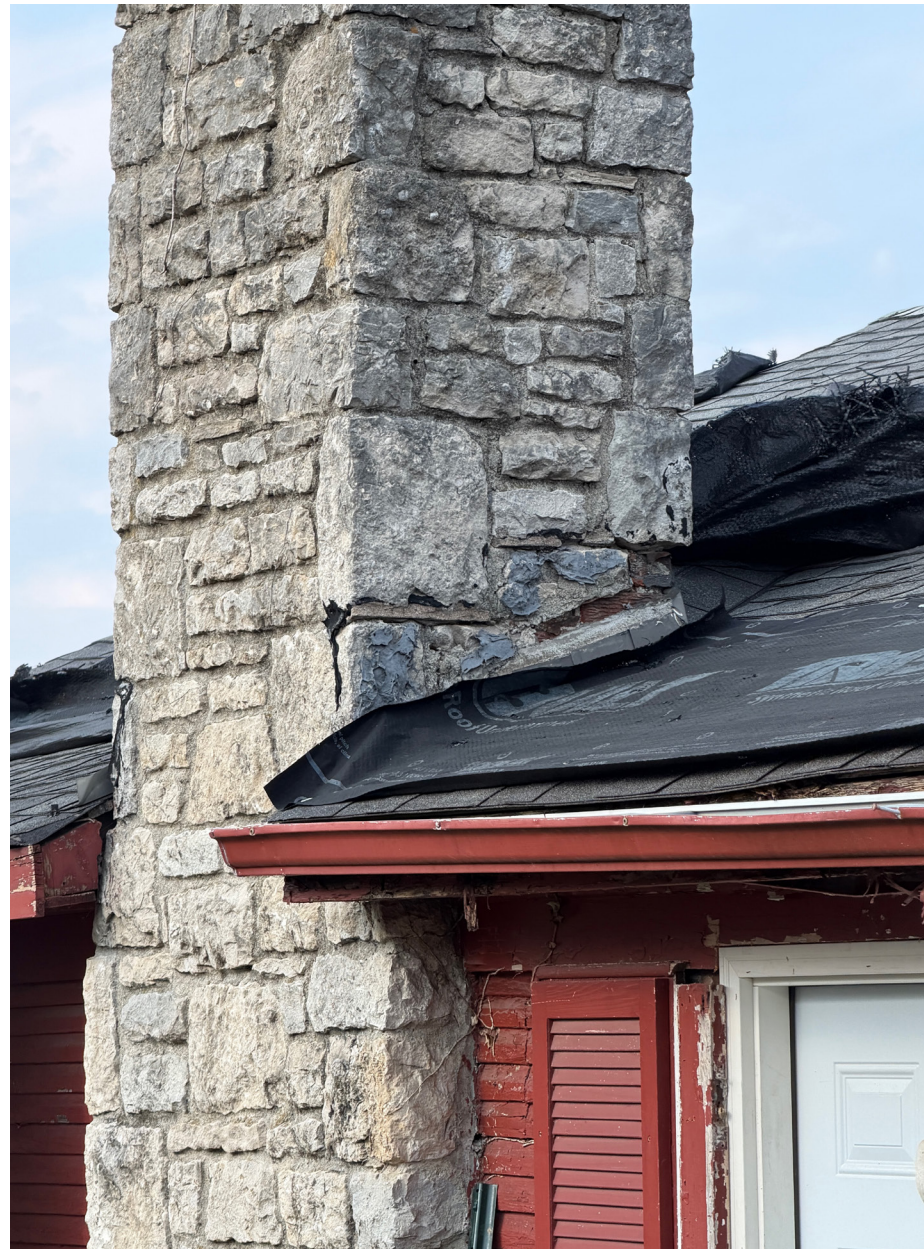
Chimney Detail, showing Brick under Stone
