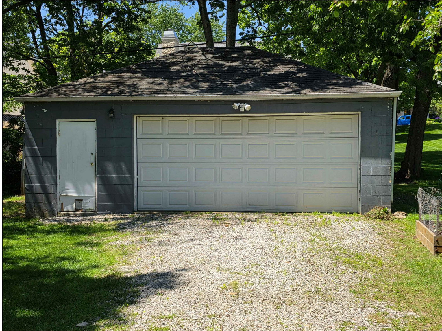
existing garage before
