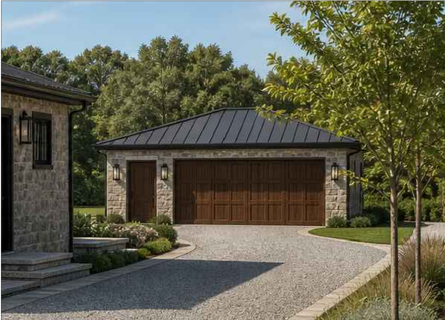
existing garage after
