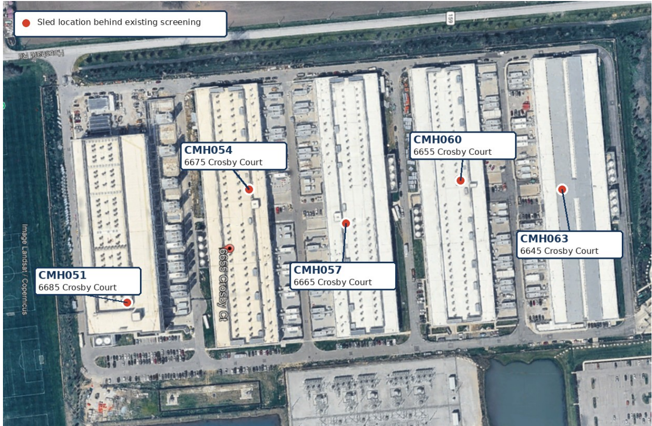
Figure 1 Updated sled locations behind existing rooftop screening
