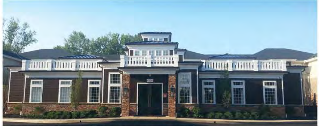
Vinyl Windows Single Hungs and Patio Doors – Palmer House (Clubhouses for both are Premium Painted vinyl), by Preferred Living NEW ALBANY
