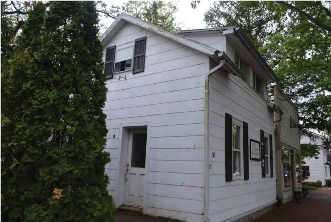
Photo 5- The cabin has little activation of the street edge, only two small windows. The entry is removed from the street on the North of the building.
