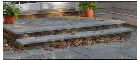
Porch Construction Style Random Rect. Bluestone with Fieldstone Risers and Wall
