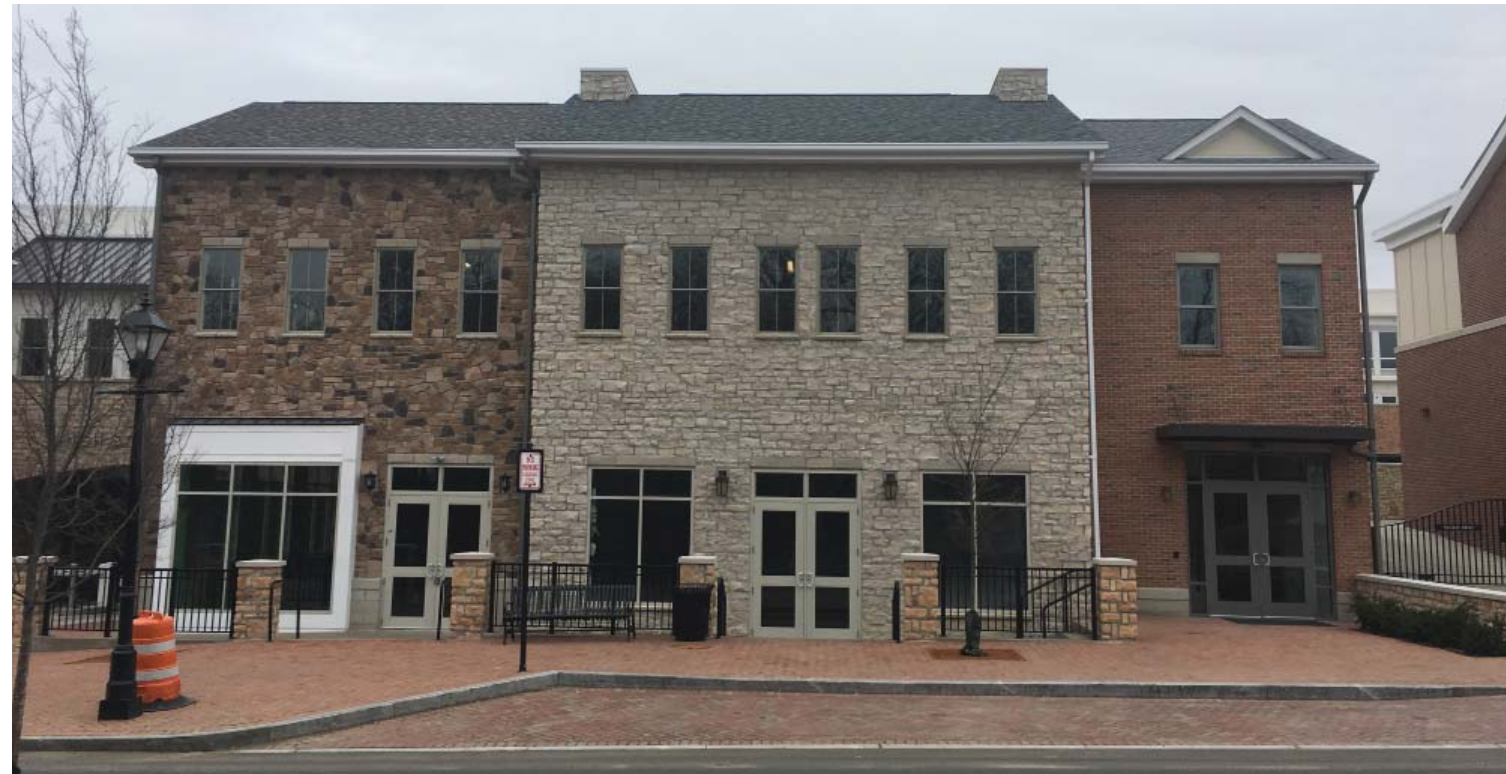
EXISTING NORTH HIGH STREET FACADE
