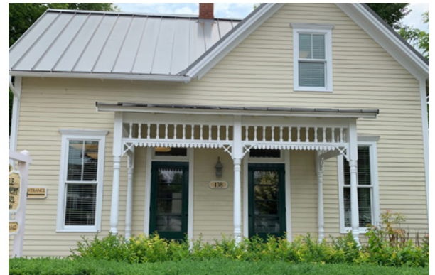
Original architectural details, 138 South High Street
