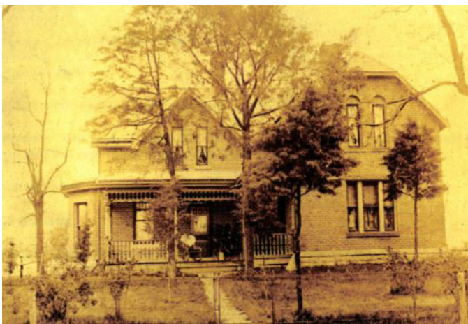
167 South High Street, built 1897 in the Queen Anne style. Elements of the style include the asymmetrical massing, irregular floor plan, bay windows, decorative gable ends, wrap-around front porch with decorative spindle work, and decorative shingles in the roof.
