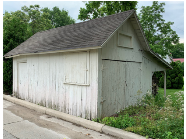
Historic outbuilding, 83 South Riverview Street
