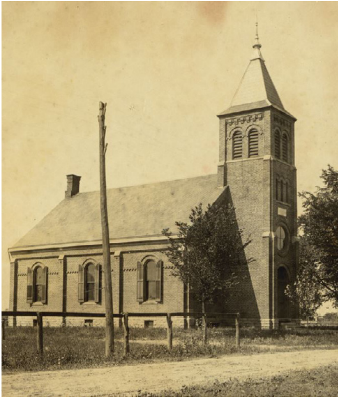
St. John Lutheran Church at 6135 (6115) Rings Road, built ca. 1860, is an example of Romanesque Revival architecture. Note the Romanesque Revival-style elements such as the masonry construction, round arches, brick corbeling, and square tower.
