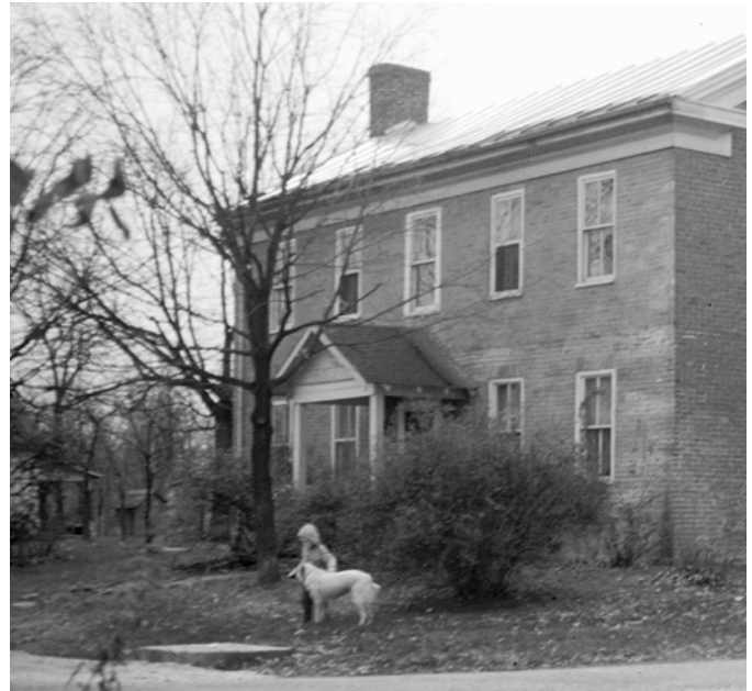
109 South Riverview Street, built ca. 1827, is an example of Federal architecture. Note the Federal-style elements such as the two-story height, rectilinear form, five-bay façade composition with symmetrical window and door placement, and a side-gable roof.
