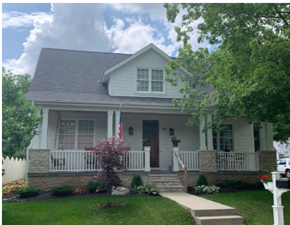
Finished foundation, 73 South Riverview Street
