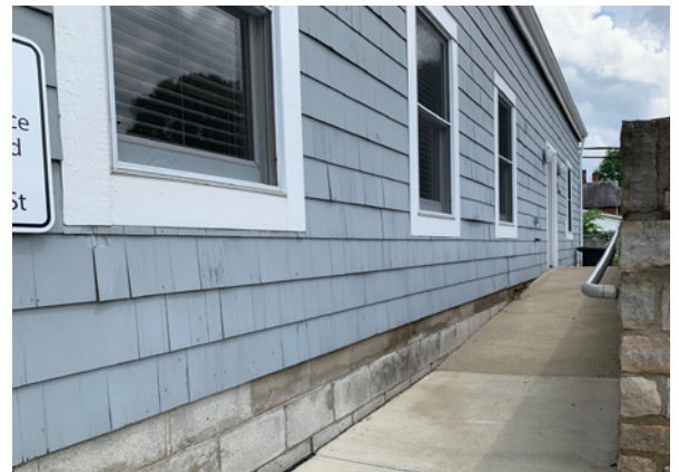
Rear ADA ramp with masonry wall, 129 South High Street
