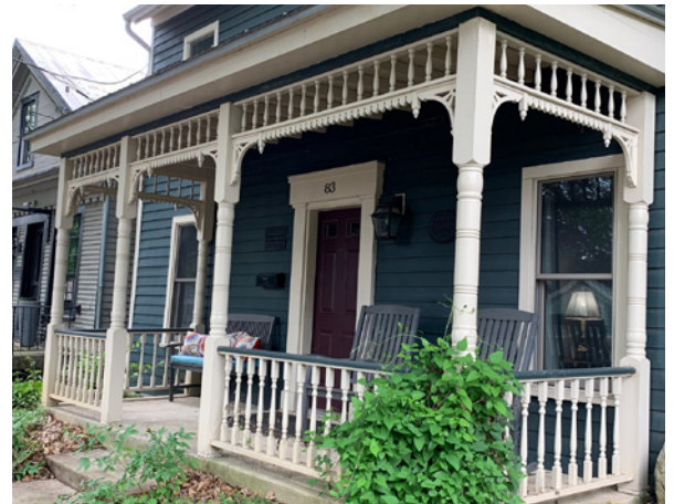
Original porch, 83 South High Street
