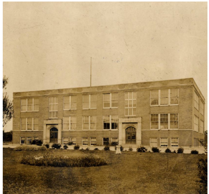
The Washington Township Centralized School at 150 West Bridge Street, built in 1919 in the Art Deco style. Elements of the style include the smooth wall surface and decorative concrete panels with stylized or geometric motifs.
