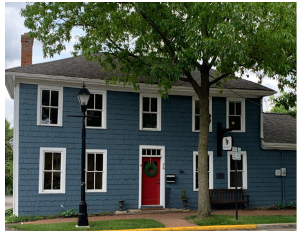
Historic building color, 76-78 South High Street
