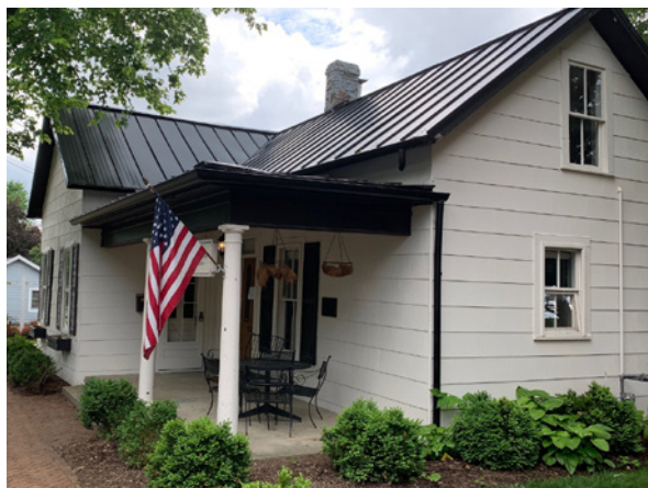
Historic building color, 113 South High Street
