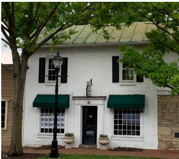
Commercial storefront, 14 South High Street
