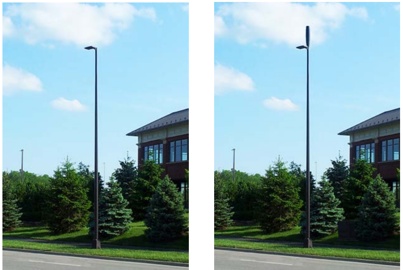
Figure 5.5A--Illustration of Collocation on Existing Standard Light Pole with Ground Mounted Facilities Cabinet Integrated into Existing Landscaping
