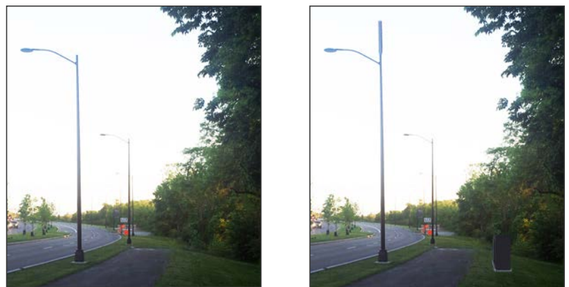
Figure 5.2C--Illustration of Type 1 Collocation with Ground-mounted Small Cell Equipment along Open Space within the Right-of-Way.
