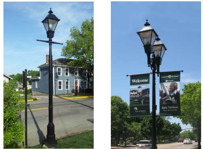
Figure 5.1C--Decorative Pedestrian-Scale Street Lights in Historic Dublin
