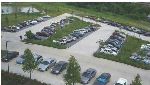
Parking lot stormwater approach: Curb breaks to accommodate inlet flow; large central islands
