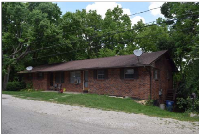
110-112 S Riverview St, looking northeast
