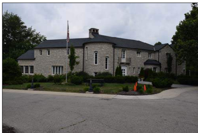
7125 Riverside Dr, looking northwest
