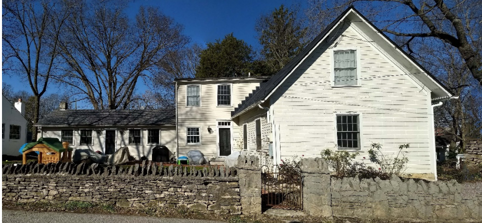
4. Panoramic photograph of the south side of the current building. Note the simple gable rooflines and the edge of the existing garage to the far left of the photograph.
