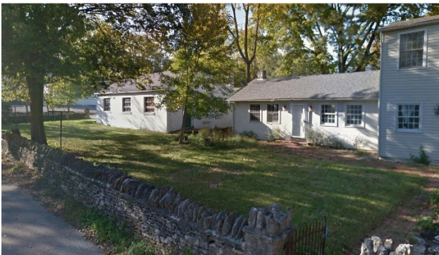
3. View of the rear of 63 S. Riverview Street with the existing one-story addition and detached garage. A second story master suite will be added to the one-story addition. (Source: Google Earth).
