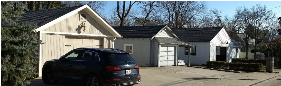
Row of existing garages along Blacksmith Lane. The current garage at 63 S. Riverview Street is to the far right. Note the size, scale, and features of the garage structures. In its current form, the proposed garage addition will overpower the existing ones and detract from the overall historic district.
